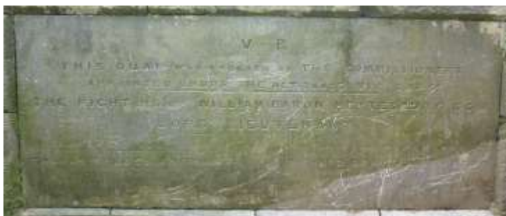
Plaque of wall of quay, Clarecastle – photograph courtesy of Eric Shaw
